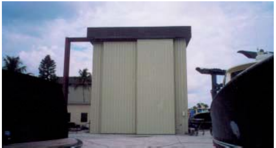
The Hinckley Yacht facility in Stuart, FL, is closed by a Well Bilt rolling door.
