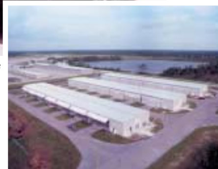
These hangars feature bi-fold doors from Well Bilt Industries.
